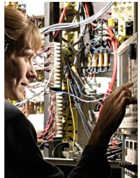
Multi-Phase Marine Converter Testing
